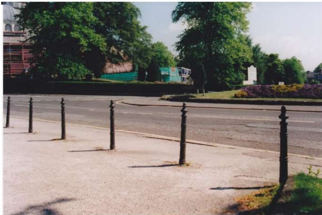
Bollards, St. John's Church Six cast iron bollards to the east of the church.
